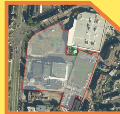
Figure 1: Kingsway Quarter site boundary
