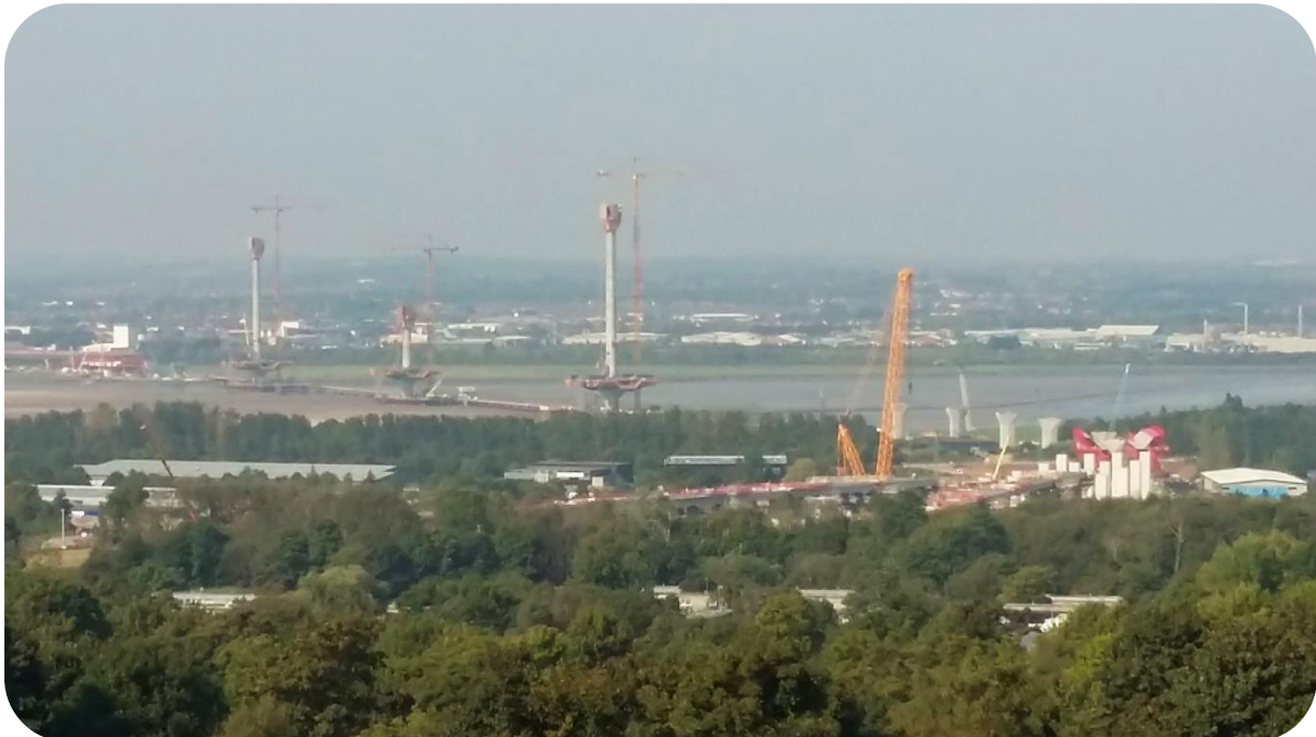
Figure 8.2 – Photograph showing Mersey Gateway construction
