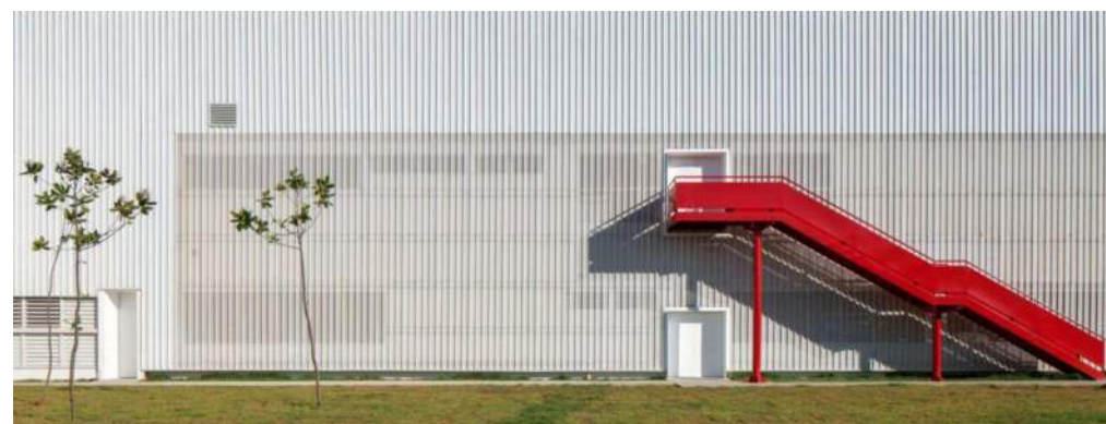
Using colour to add interest to otherwise blank facades: Knorr-Bremse factory, São Paulo
