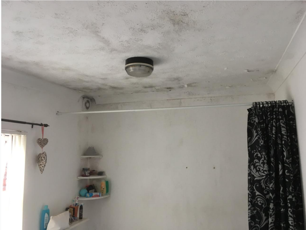
Damp and mold in kitchen and bathroom
