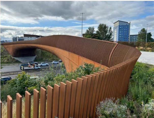
↑ Sighthill, Glasgow. Bridge providing direct pedestrian and cycle access across the M8 motorway, utilising an organic architectural form and soft landscaping, creating an iconic structure and celebrated connection to a developing neighbourhood.
