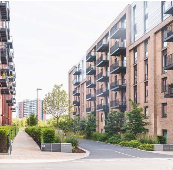
↑ Middlewood Locks, Salford. Verdant planting, sustainable urban drainage, on-street car parking and generous and direct pedestrian routes. The streets here allow for all movement types, but do so in a manner which treats the streets as green streets, calming and softening the environment and benefiting the wider public realm.
