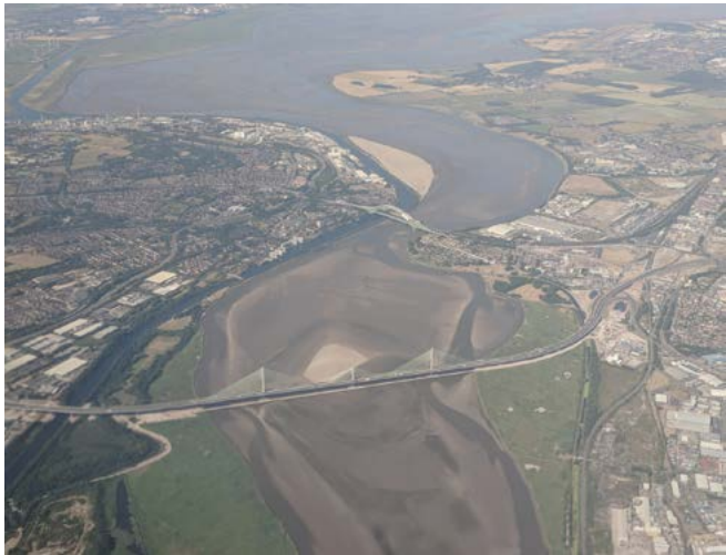
Mersey Gateway bridge and Halton bridges
