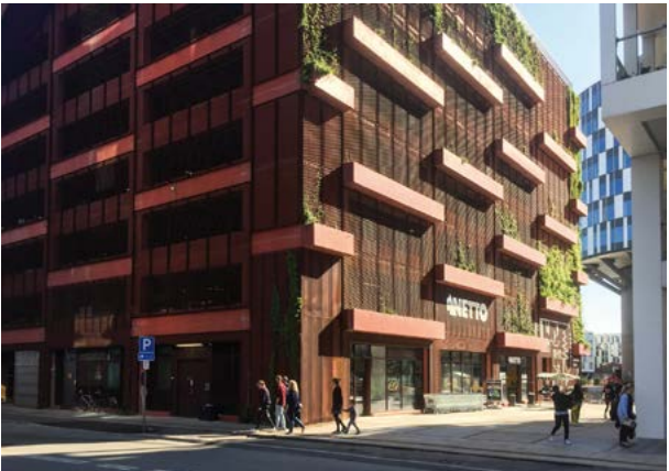
↑ Nordhavn car park, Copenhagen. This offers a centralised 'mobility hub' at the centre of a neighbourhood. The building provides car parking, as well as a supermarket, cycle parking, cycle hire, and a play facility for all ages on its rooftop, providing a multi-functional facility and highly efficient use of land.
