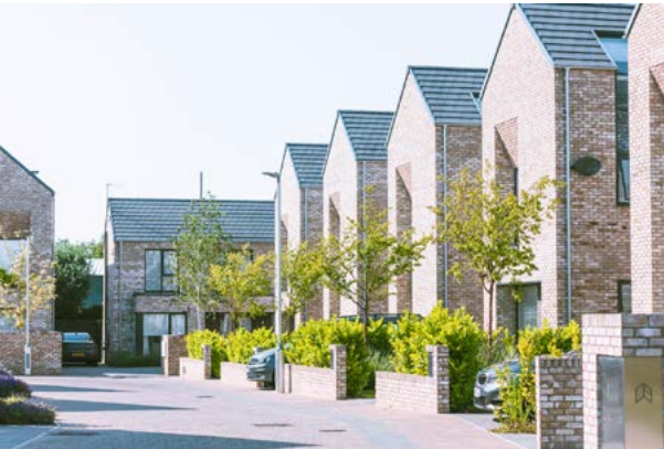
◀ Goldsmith Street, Norwich. ▲ The Gables, Crosby. High quality urban family homes.
