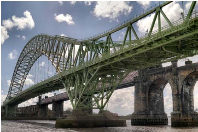
Runcorn railway bridge and Jubilee bridge from Victoria Gardens
