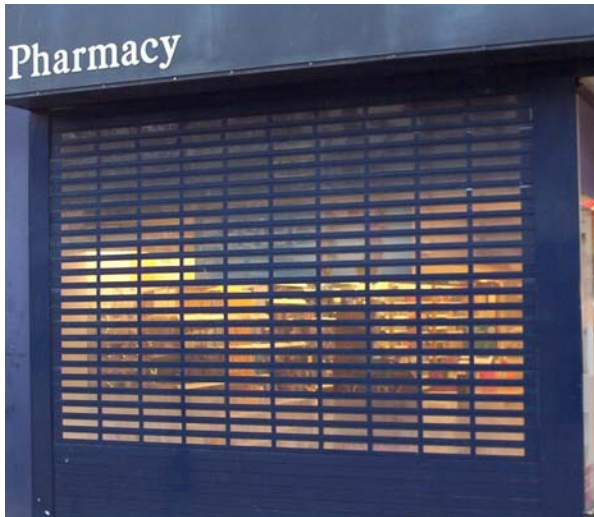
Photo 7: Good example of shutter use, where the interior of the shop is still visible and can continue to add to the street scene, and the shutters are painted to complement the rest of the shop unit.
