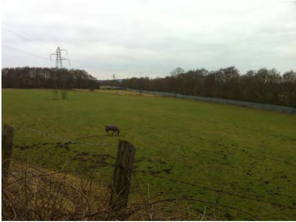
Pylons and overhead power lines crossing the site
