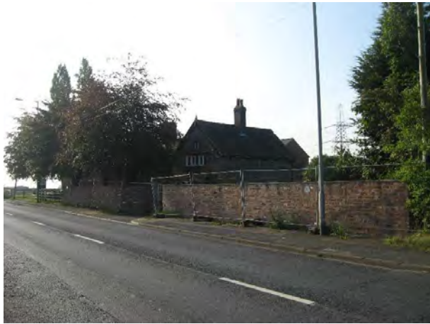
View of Sandhills Farm Buildings
