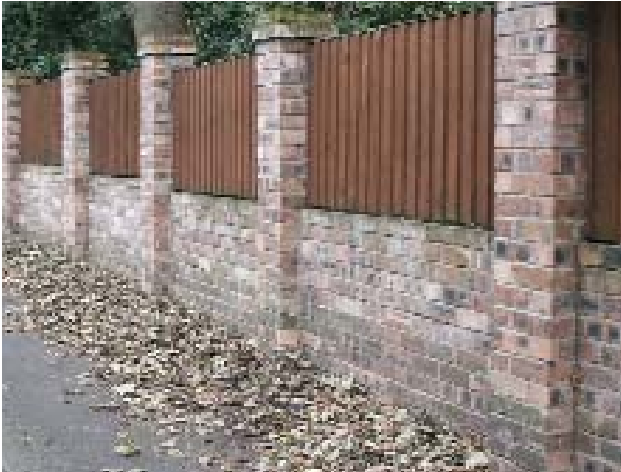
Brick wall combined with wooden fencing provides durable boundary treatment but reduces natural surveillance.
