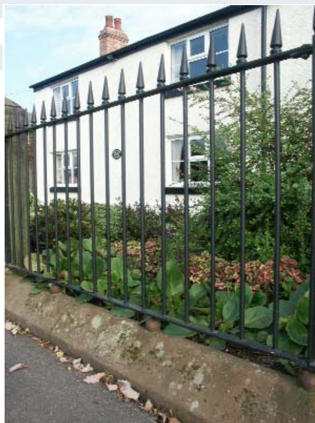
Ornate railing within a conservation area provide security, opportunity for surveillance and are sympathetic to their surroundings.
