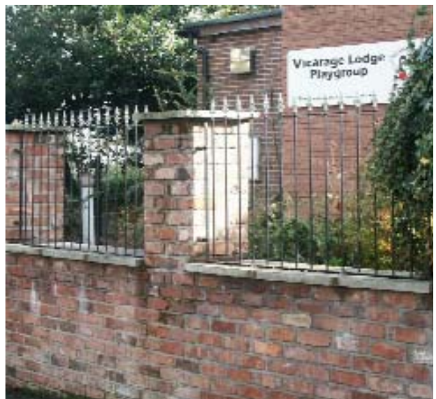
Combining brick and railing provides an attractive and secure boundary which provides opportunities for natural surveillance.
